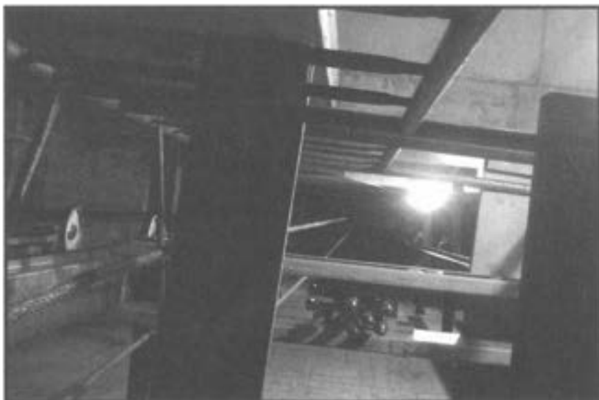
Some elevator shafts, such as this one under construction, provide ladders for easy climbing.
