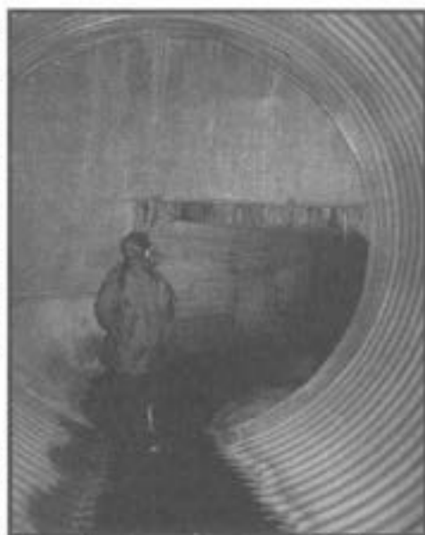
Many drains contain interesting changes in shape and construction material.
