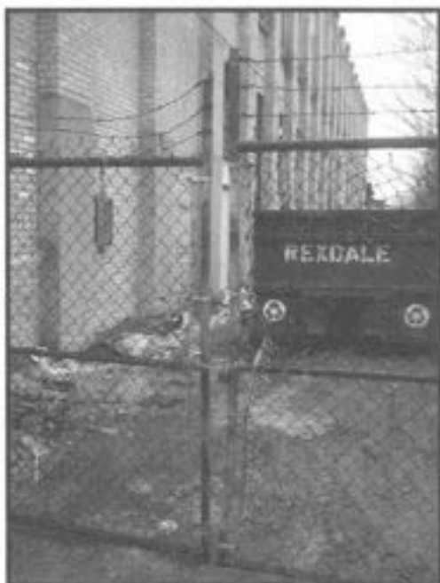
Loose barbed wire poses less of a threat than tightly stretched barbed wire.
