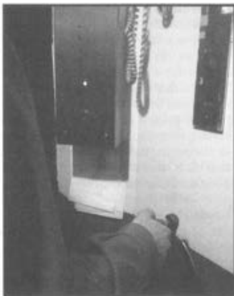
Older, cooler elevators may lack up and down buttons and instead have one lever that controls speed and direction.
