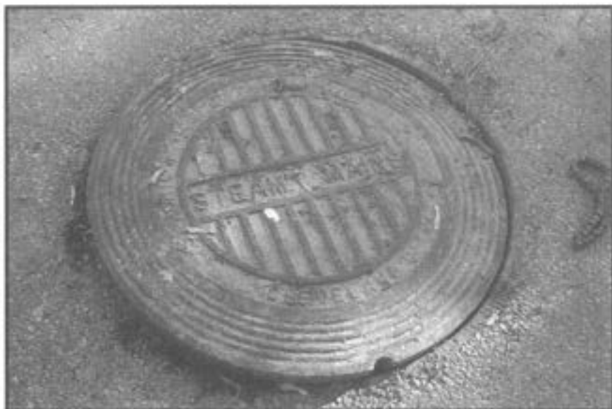
Sometimes the entrance to the utility tunnel system is obvious.
